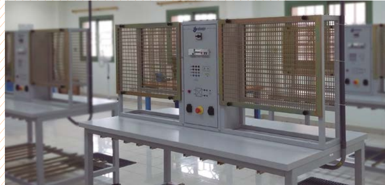
Electrical Installation Laboratory. COE MUHAYIL – ARABIA SAUDI
